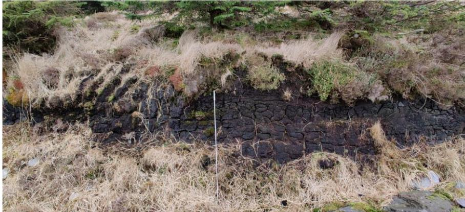
**Figure 3-3: Compact peat side-cast along a track during previous construction works.**
